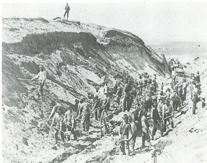
The Big Cut. Northern Pacific Railroad original construction in 1879.
