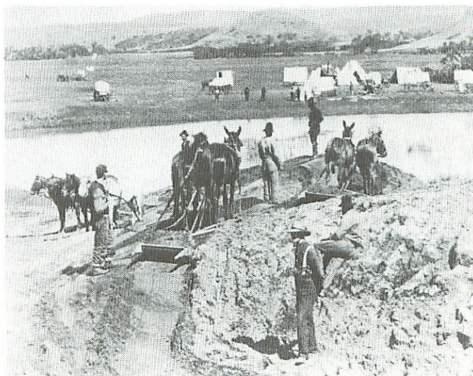
Sweet Briar Valley, Dakota Terr. Northern Pacific Railroad construction crew in 1879, grading in advance of track laying. (At this time, track work was delayed west of Bismarck.)
